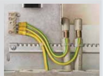
Shield connection with SA KRF
