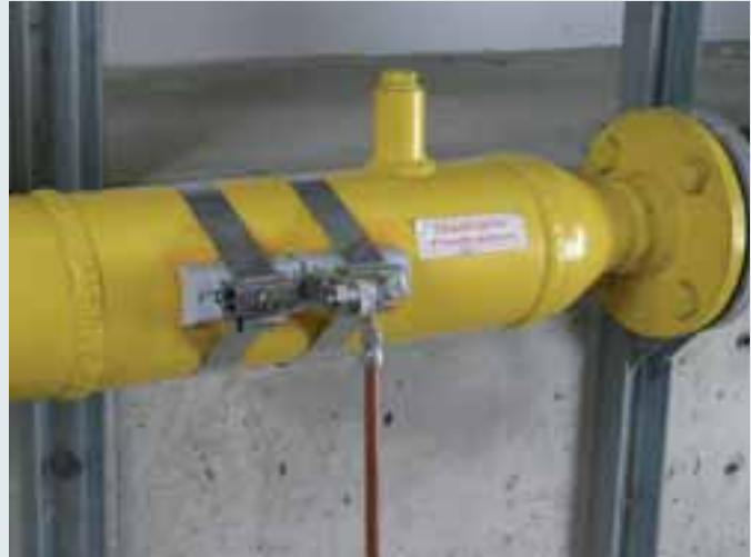
Pipe clamp for attaching to pipes in hazardous areas for lightning equipotential bonding according to EN 62305-3 (DIN VDE 0185-305-3)
